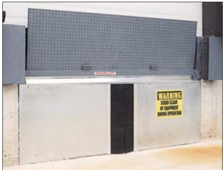
Pentahook in stored position, ready to accept truck.
