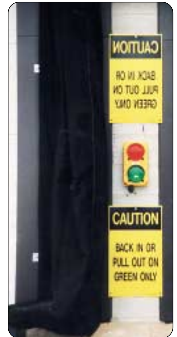
Exterior Communication System (view from truck mirror)
