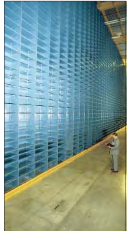
40' high shelving ready for loading.
